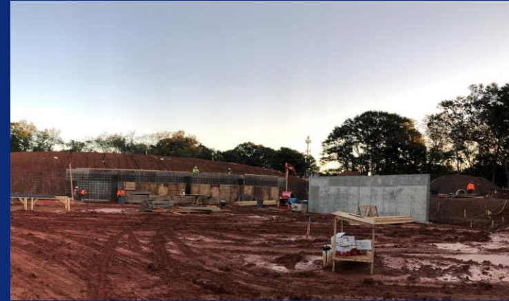
Concrete wall reinforcement and forming at north wall of gymnasium
