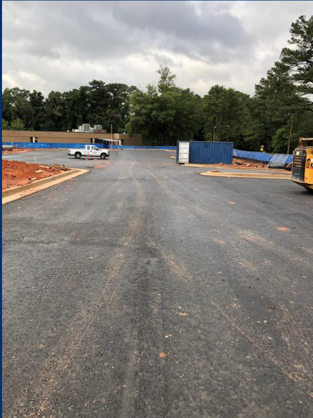
Binder course laid in parking lot and Richland Road cut through
