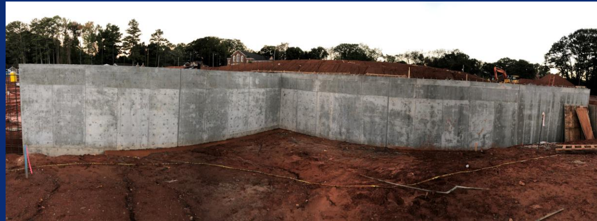
Poured reinforced concrete wall at southeast corner of building
